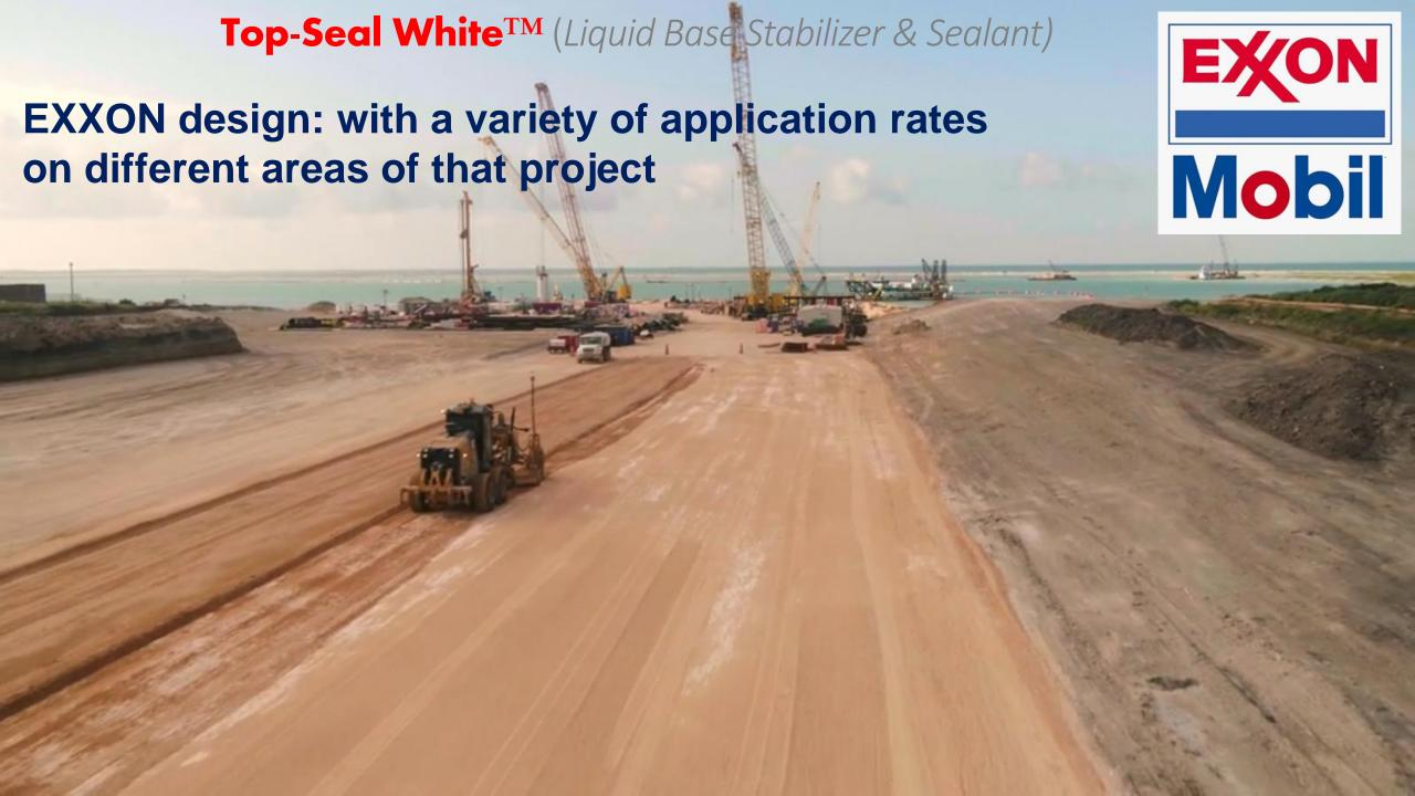
Exxon road design for heavy haul road (HHR) supporting up to 140psi SPMT wheel loads.
