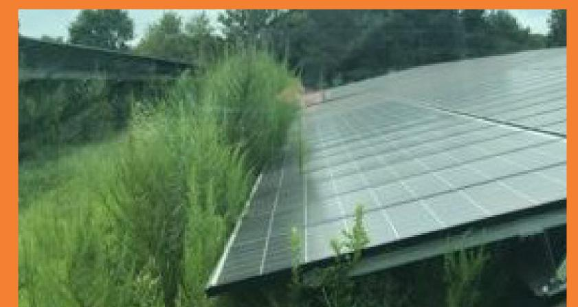
Because the soil stabilizer behaves as pavement, we believe it will block vegetation growth where it is applied: possible savings in maintenance costs
