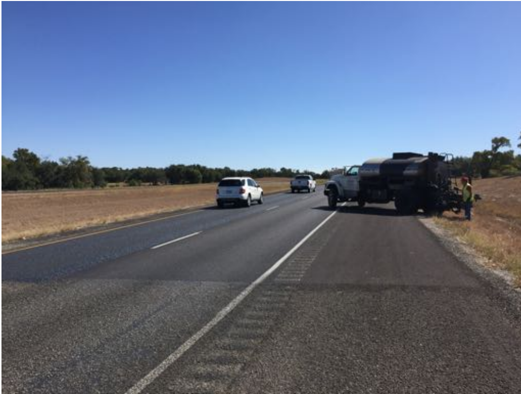
Picture 1: The starting point of the pavement (an asphalt emulsion based fog seal was applied previously to the left lane)
