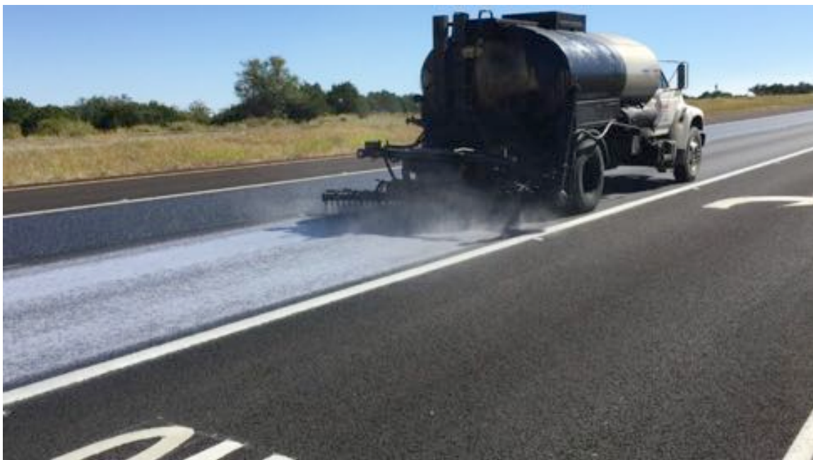
Picture 2: The shot was little less than 0.15 gal/sy. This provided good coverage without runoff.
