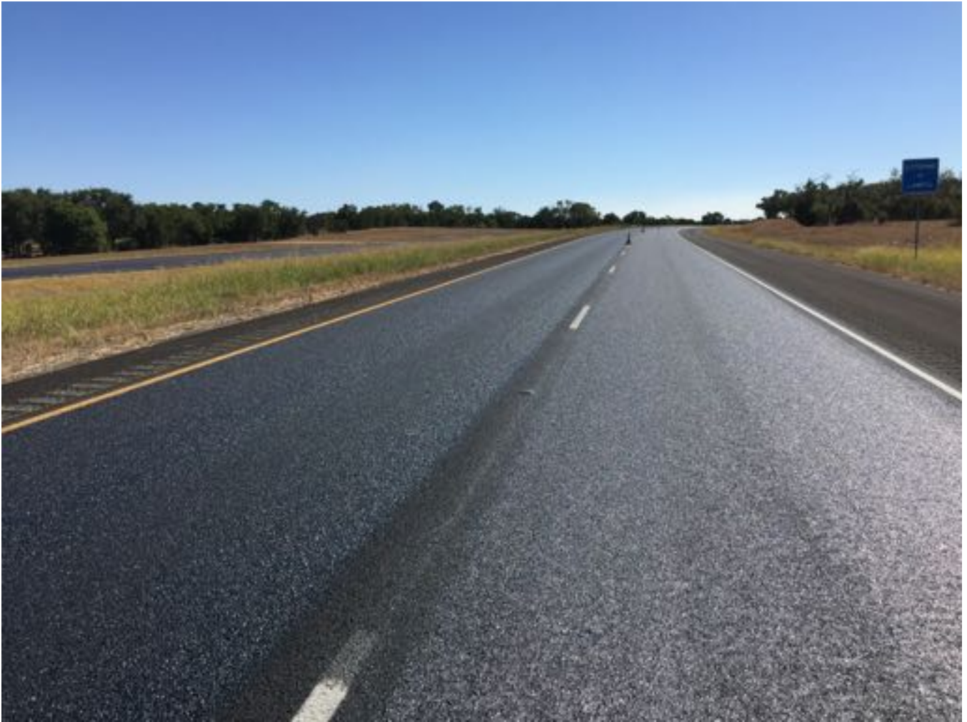
Picture 4: There was literally no runoff onto the striping and excellent coverage of the aggregate was achieved.
