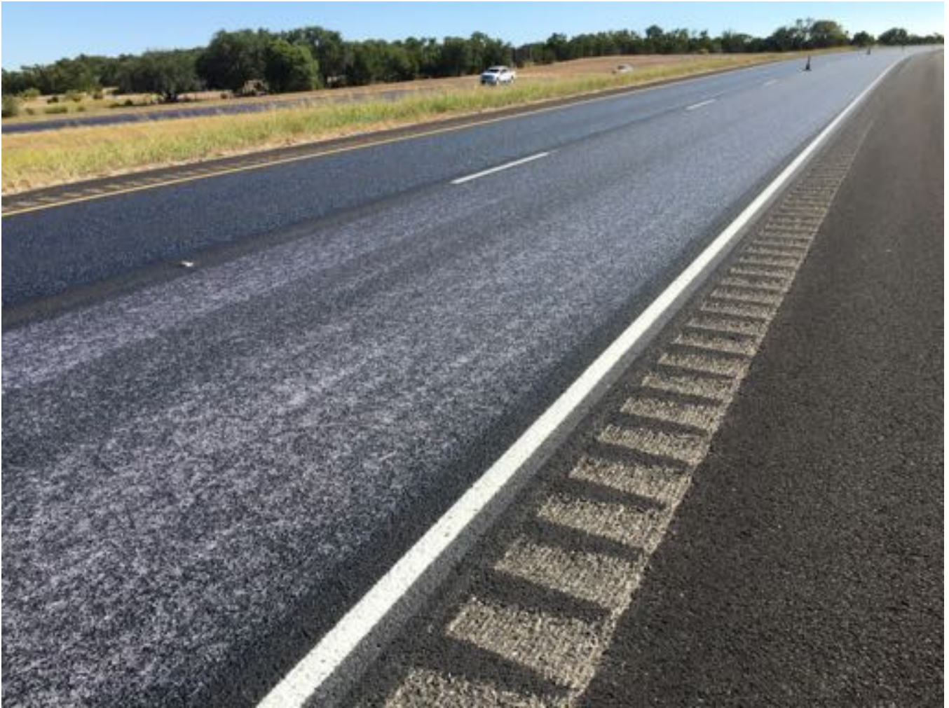
Picture 3: Just after the application, the color is light gray and gets darker as curing occurs only by evaporation of water.
