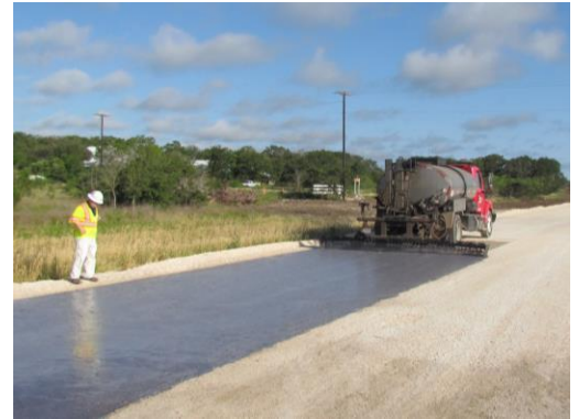
Terra Prime™ application in Florence, Texas
