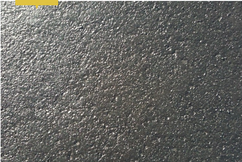
RESULT | TSB close-up after 48 hrs of curing time
