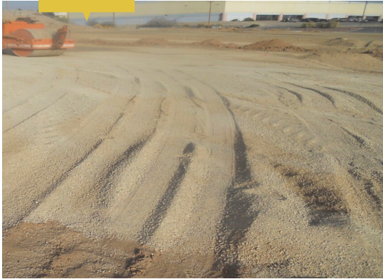
Loose soil prepared for application of TSW
