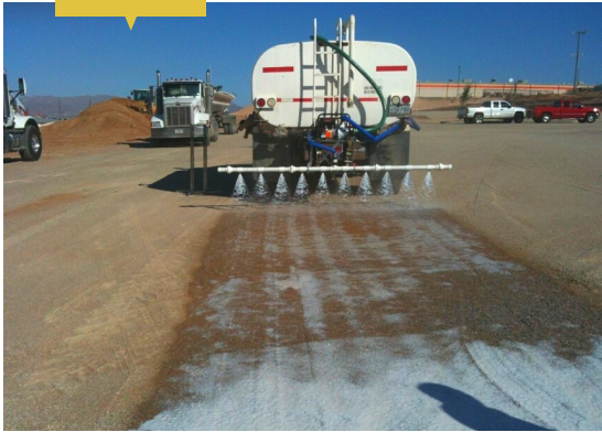
First application of TSW
