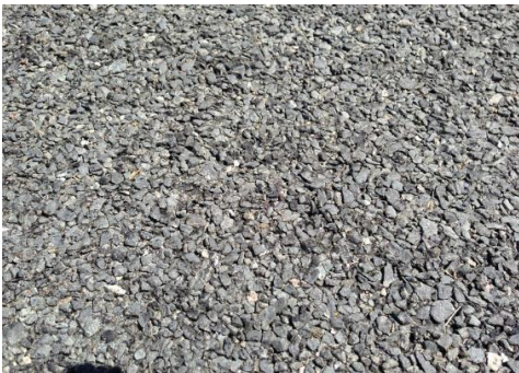
Before Application with Terra Fog™
