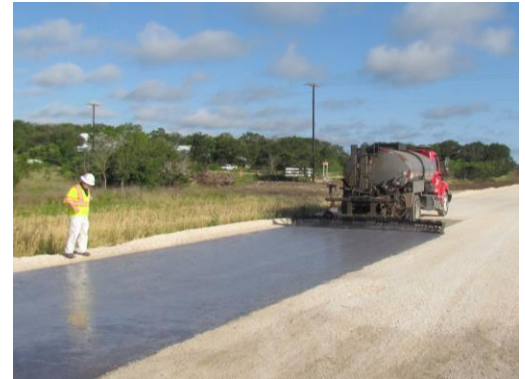
Terra Prime™ application in Florence, Texas
